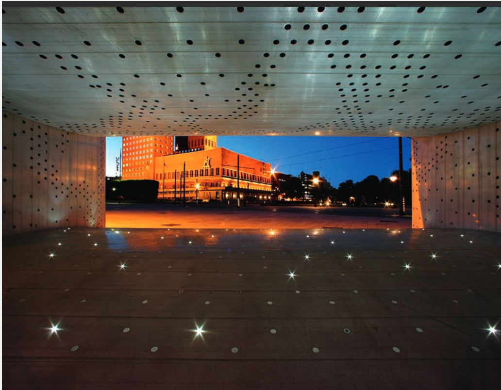
Construction – canopy manufactured with FSW
