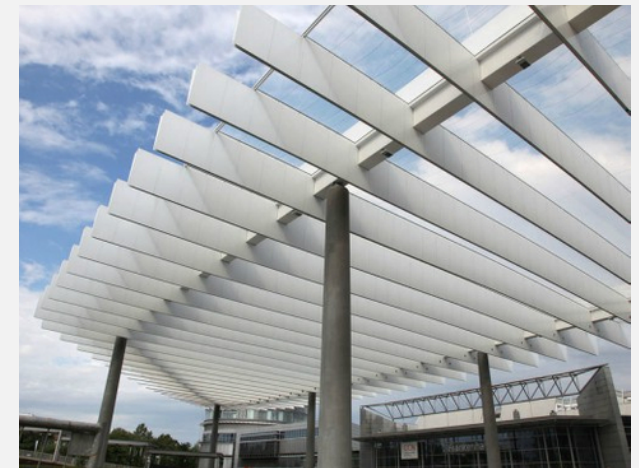
Gangway and weather shield
